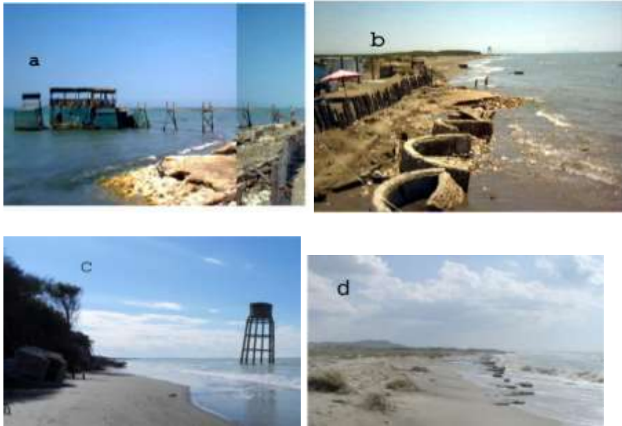
Fig.2: Semani beach: (a) concrete borehole basement; (b) beach view from the bridge; (c) submerged water tower; (d) shore abrasion in Qerreti beach.
