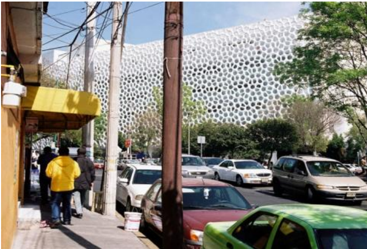
Fig. 5: Facade that eats smog, Hospital in New Mexico City https://architazer.com/blog/inspiration/industry/smog-eating-facades-and-the-future-of-our-air-quality/#:~:text=The%20innovative%20technique%20has%20recently,TiO2%20developed%20by%20Elegant%20Embellishments
