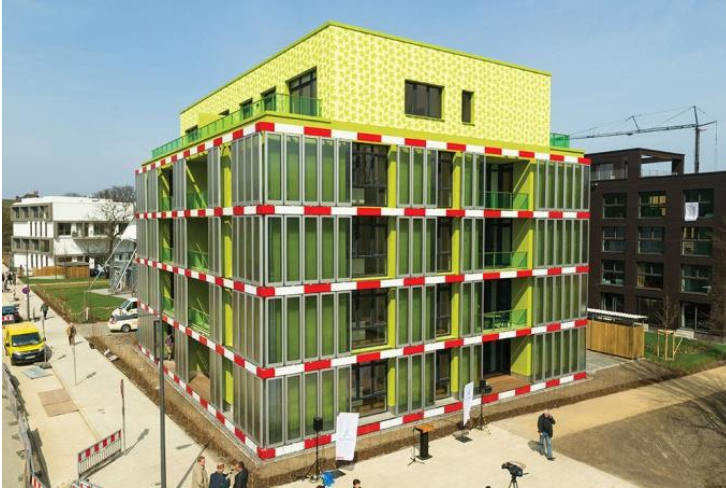
Fig. 3 Energy producing algae facade(futher information could be found in http://www.morethangreen.es/en/solarleaf-solar-leaf-algae-bio-reactive-facade/ )
