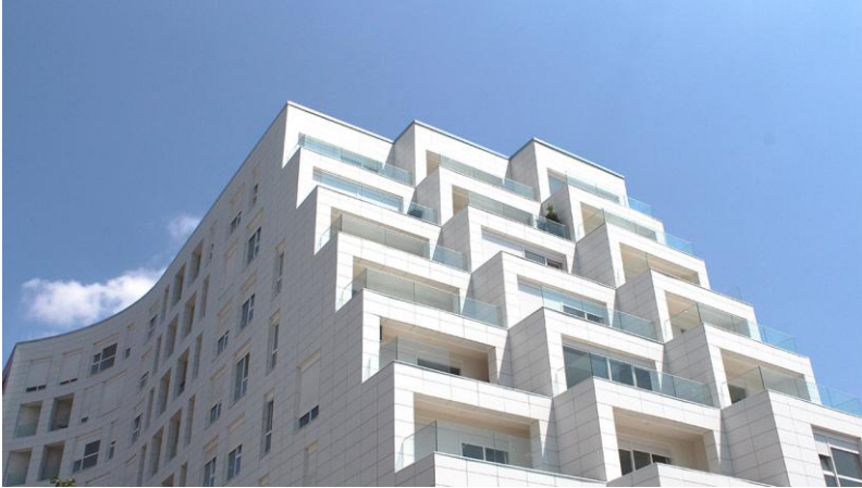
Fig. 7: Building with ventilated facade in Tirana.
